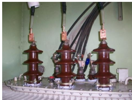
Gambar 2.13 Bushing Transformator
