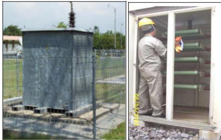
Gambar 2.26 *Neutral Grounding Resistor (NGR)* <sup>5</sup>
