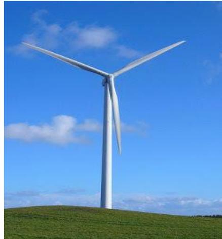
**Gambar 2.6** Turbin Angin Sumbu Horizontal
