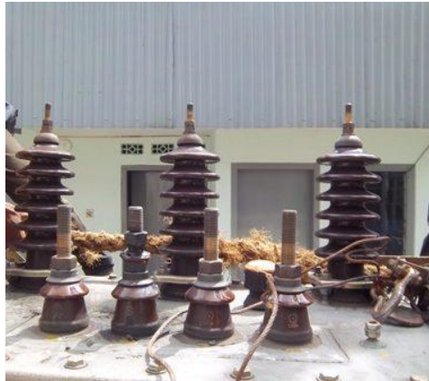
Gambar 2.9 Bushing Transformator
