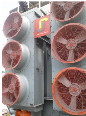
Gambar 2.11 Pendingin Transformator
