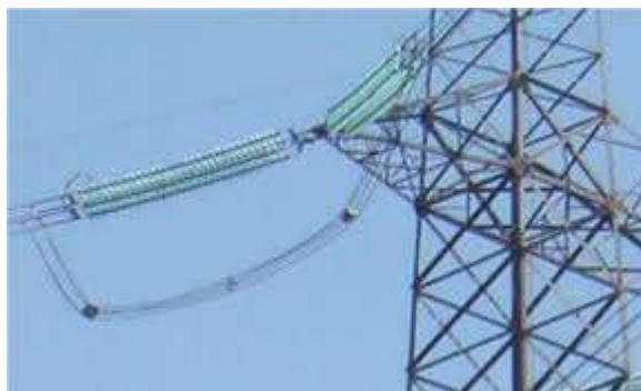
Gambar 2.18 Jumper Conductor
