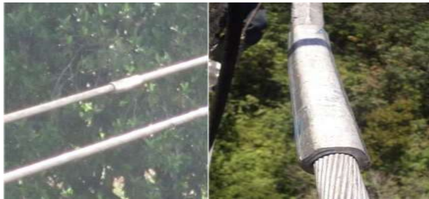
Gambar 2.38 Repair Sleeve
