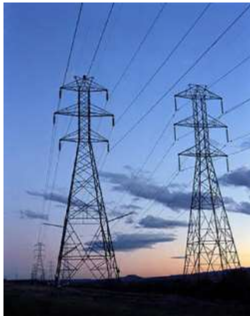
Gambar 2.32 Tiang Suspension
