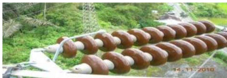
Gambar 2.24 Isolator Horizontal String
