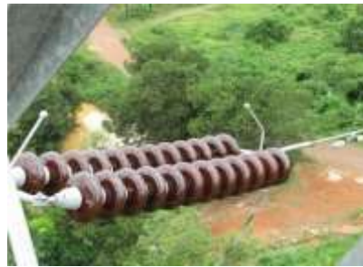
Gambar 2.28 Isolator Keramik
