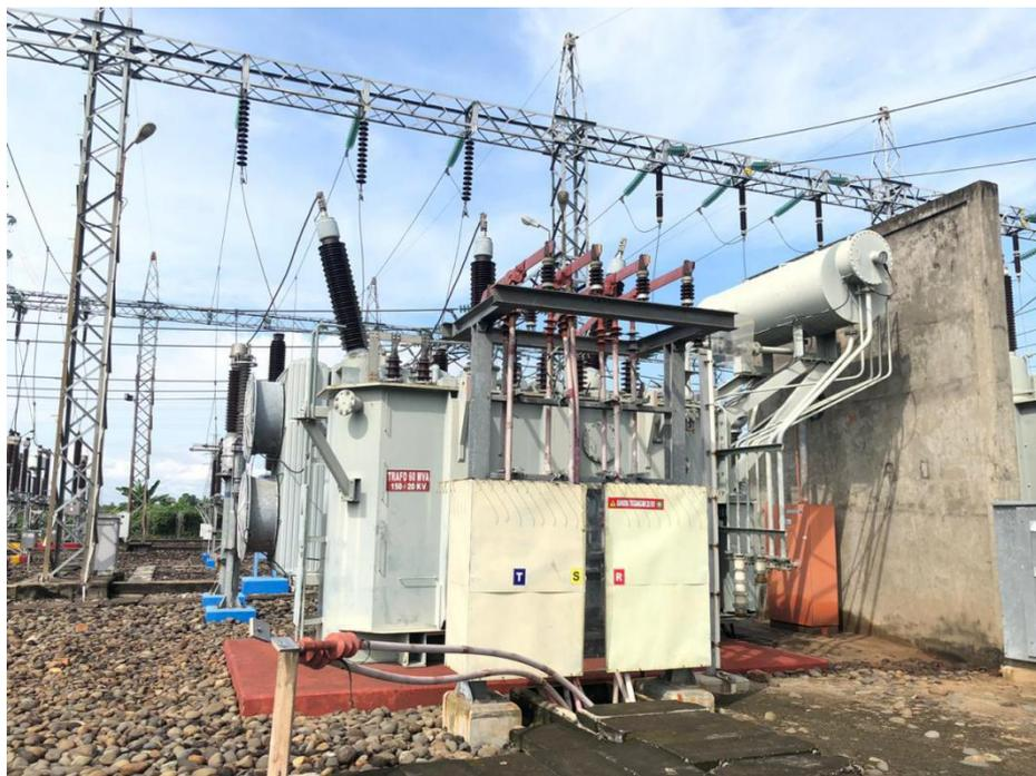
Gambar 2.2 Transformator Daya
