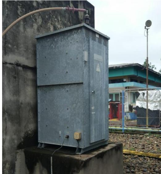
Gambar 2.12 Neutral Grounding Resistor (NGR)
