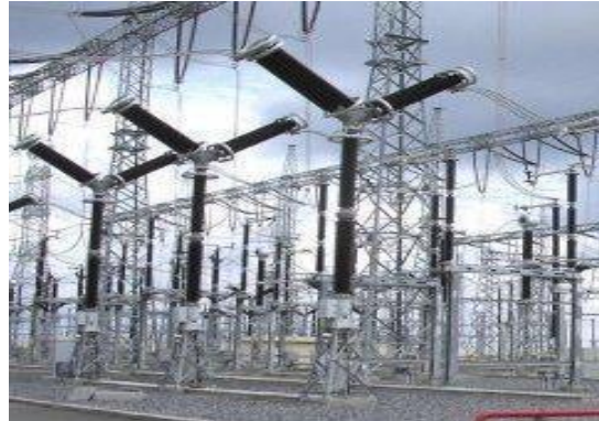
Gambar 2.9 SF6 Circuit Breaker
