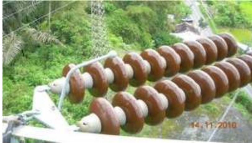
Gambar 2.7 Isolator horizontal string
