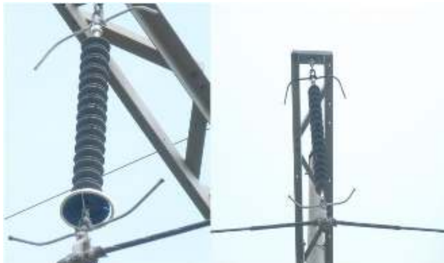
Gambar 2.4 Isolator long rod
