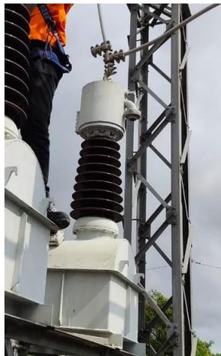
Gambar 2.1 Transformator Tegangan 70 kV
