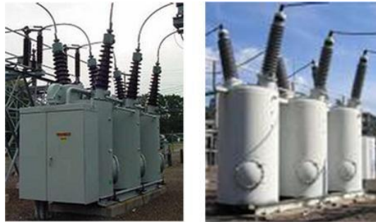
Gambar 2.9 PMT Bulk Oil
