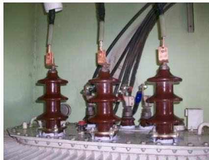
Gambar 2.13 Bushing Transformator
