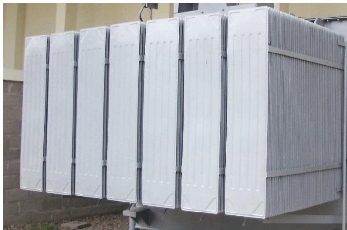
Gambar 2.15 Pendingin Transformator
