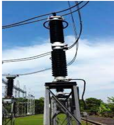
Gambar 2.8 Lightning Arrester Gardu Induk 150 kV
