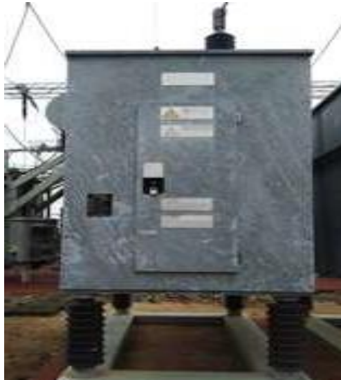
Gambar 2.12 Neutral Grounding Resistance (NGR)
