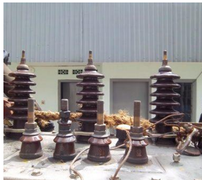
Gambar 2.9 Gambar Bushing Transformator
