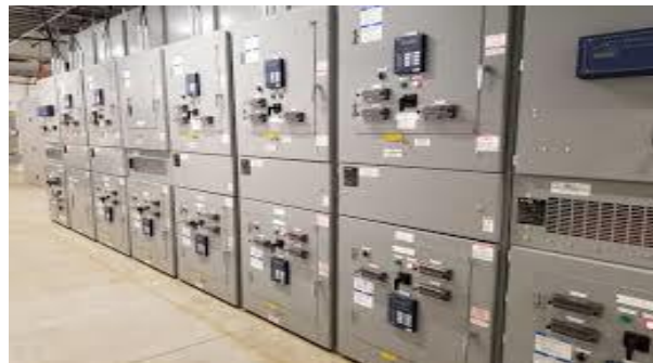
Gambar 2.1 Panel Switch Gear
