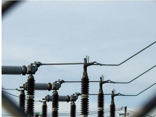
Gambar 2.6 Disconnecting Switch
