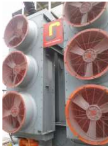
Gambar 2.11 Pendingin Transformator
