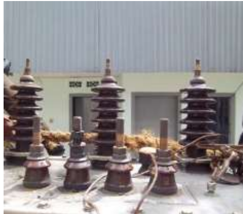
Gambar 2.9 Bushing Transformator
