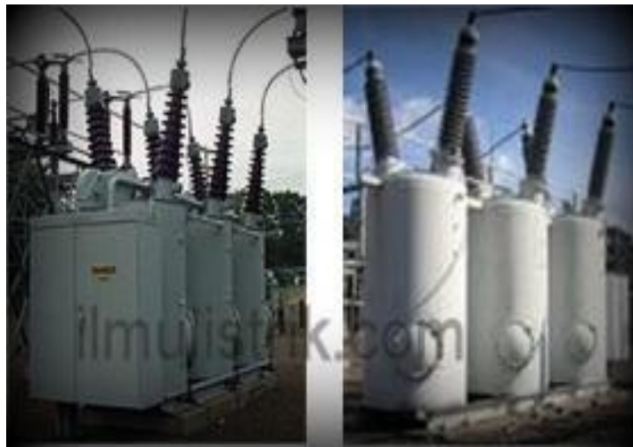
Gambar 2.5 Oil Circuit Breaker
