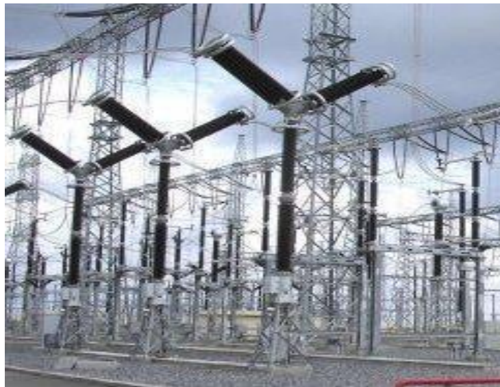
Gambar 2.9 SF6 Circuit Breaker
