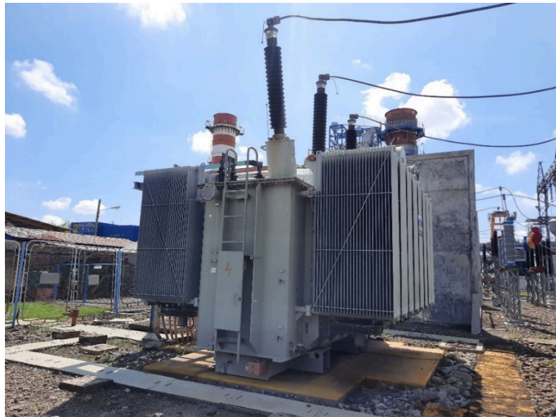
Gambar 1.3 Transformator Daya 3 Fasa 60 MVA
