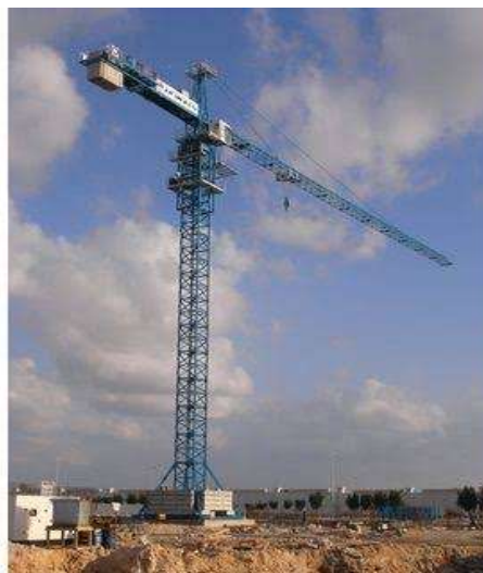
Gambar 2.1 Tower Crane (Sumber: Lit. 2, 2017)
